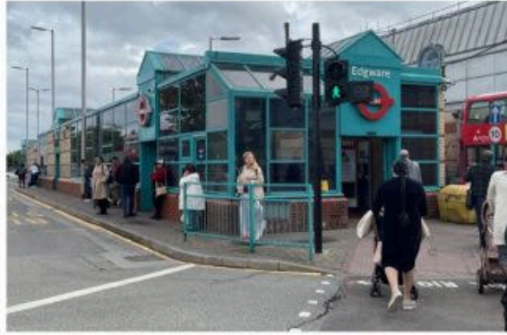
covered bus station with 5 stands
