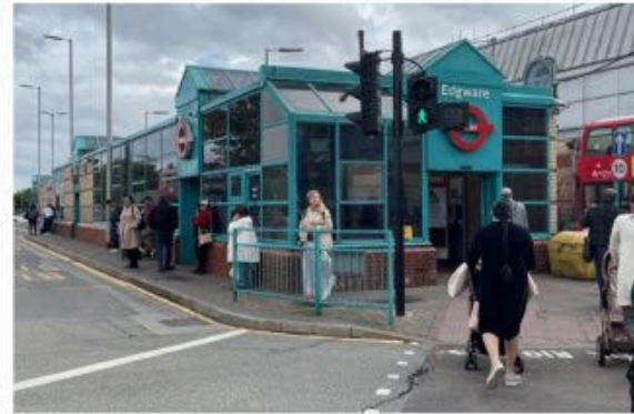
covered bus station with 5 stands
