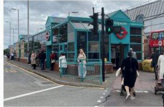
covered bus station with 5 stands
