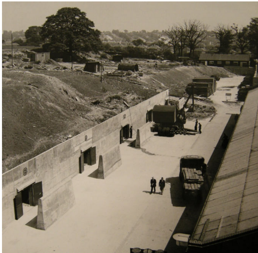
Plate 6: Air raid shelters 8 to 12 under construction (Barnet Library & Local History Centre, 1939)
