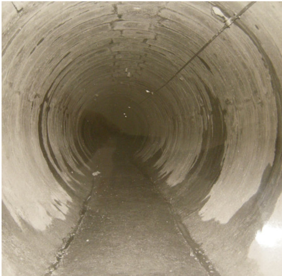
Plate 2: Completed STC Air Raid Shelter (Barnet Library & Local History Centre, February 1939)
