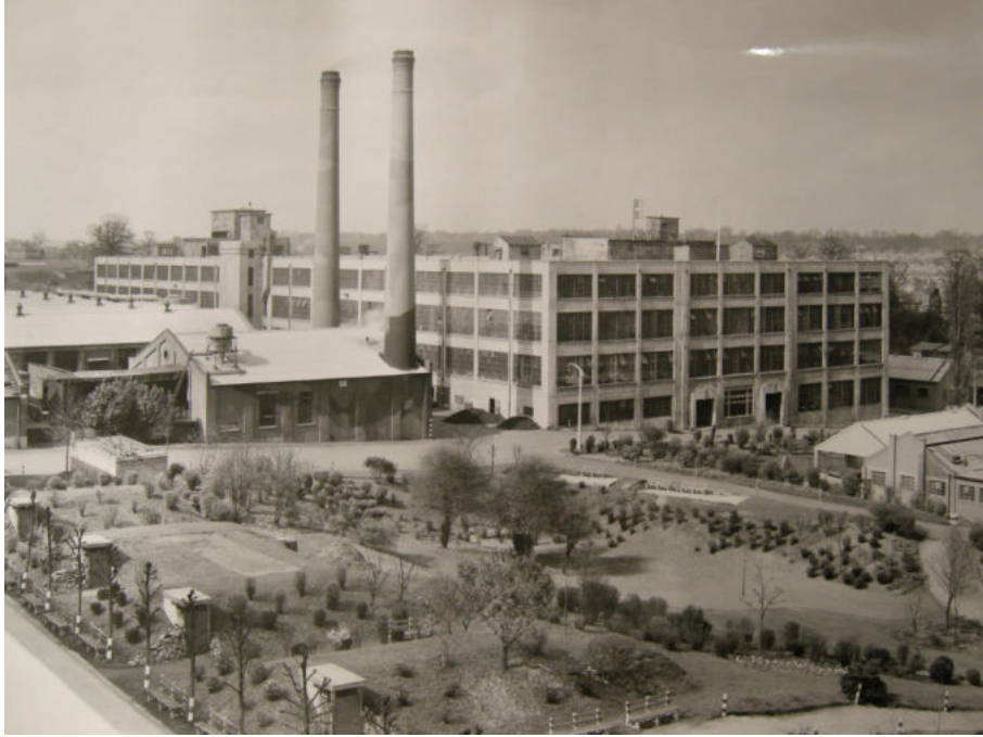
Plate 3: Post Second World War archival photograph showing air raid shelters 25 to 28; Boiler Building 10 and Building 8 in background (Barnet Library & Local History Centre)
