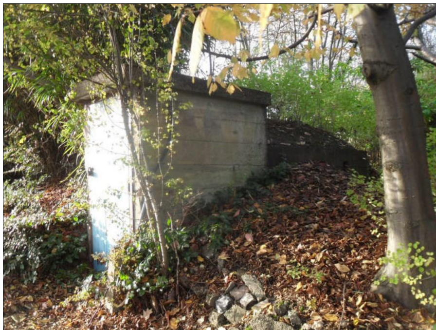
Photo 12: Extant Air Raid Shelter
