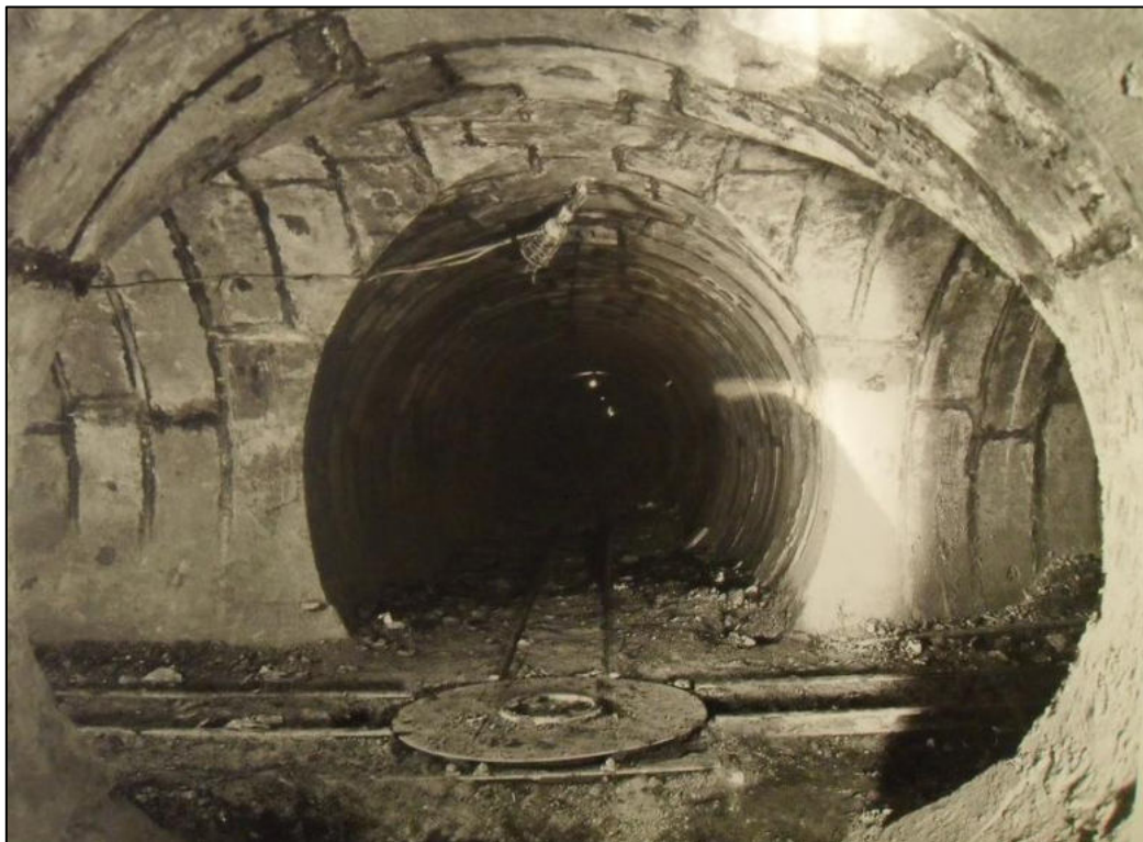
Plate 6: Underground coal chute. STC Files (Barnet Library & Local History Centre)
