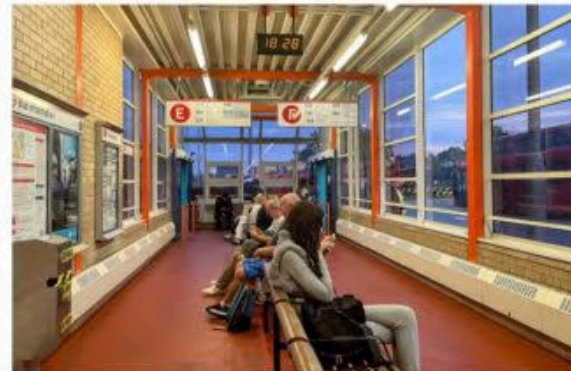
24 x 7, Safe, Well lit, Airy
