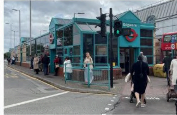
covered bus station with 5 stands
