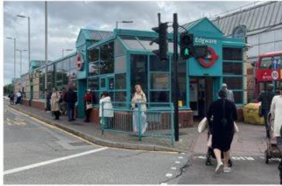
covered bus station with 5 stands
