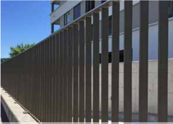
Pedestrian guardrail railings
