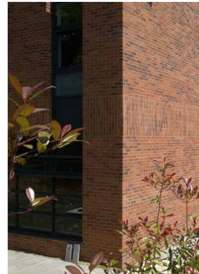
Example of variation in brick bonding
