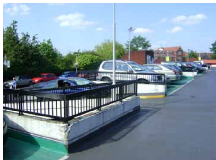
Tesco multi-storey car park
