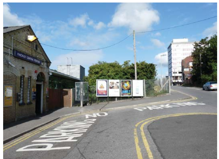
Poor sense of arrival from the station
