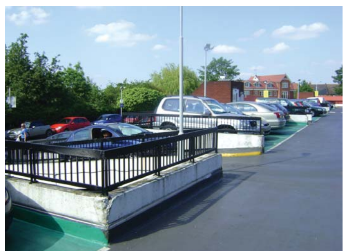
Tesco multi-storey car park
