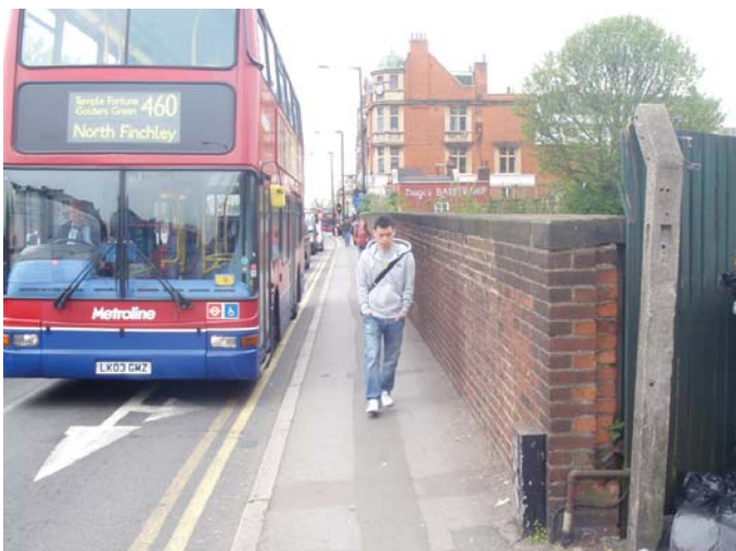
The bridge over the railway lines
