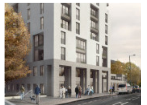
Multi-storey non-residential accommodation with residential above, Lisson Grove, London
