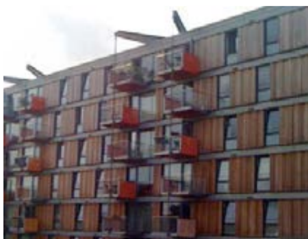
Prominent, lively frontage, Adelaide Wharf, Haggerston
