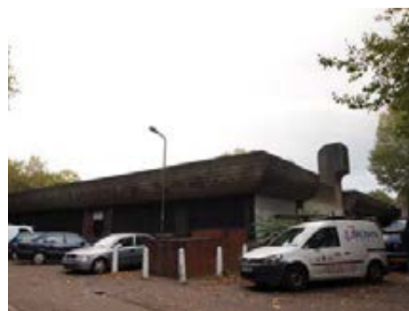
Existing energy centre
