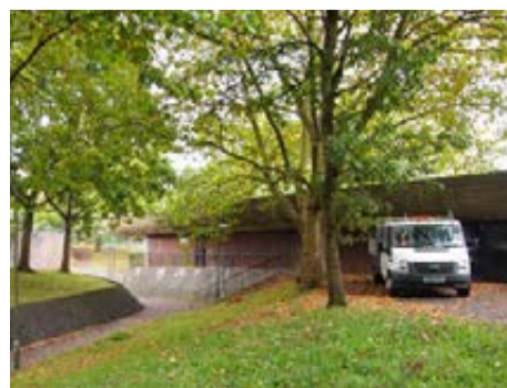
Existing energy centre
