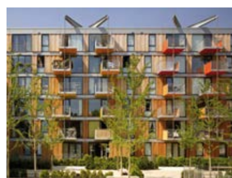
Prominent, lively frontage, Adelaide Wharf, Haggerston
