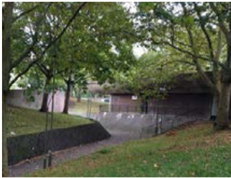
The existing sunken path leading to the energy centre
