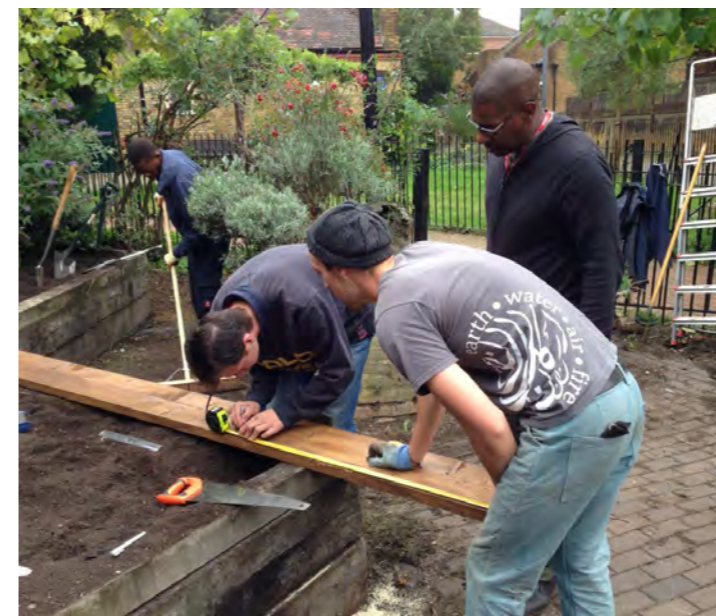
Figure 32: community construction: Time and Talents, Rotherhithe
